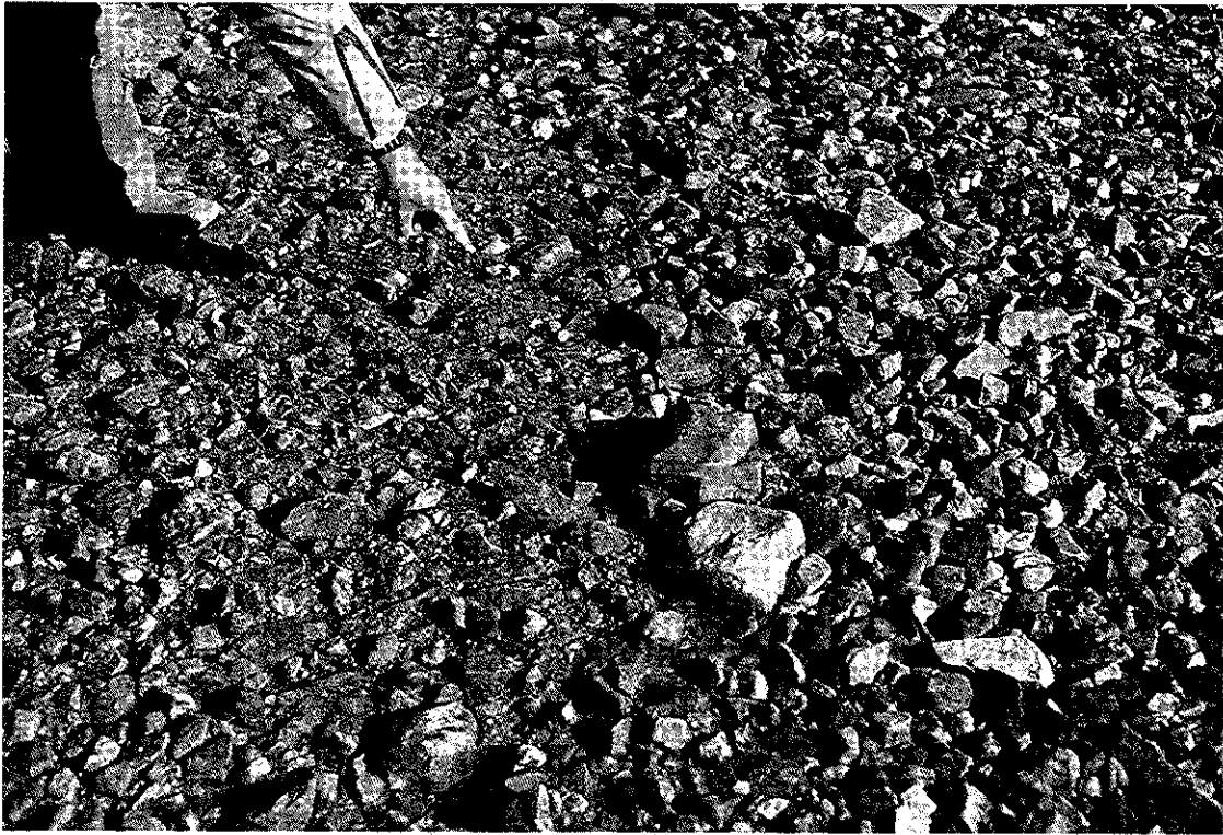
a. Bay 11 - Asphalt pavement oil/cobble/sand matrix (1989)
