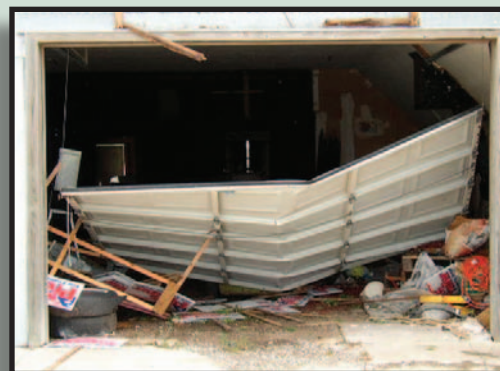
Brace garage doors from behind.
