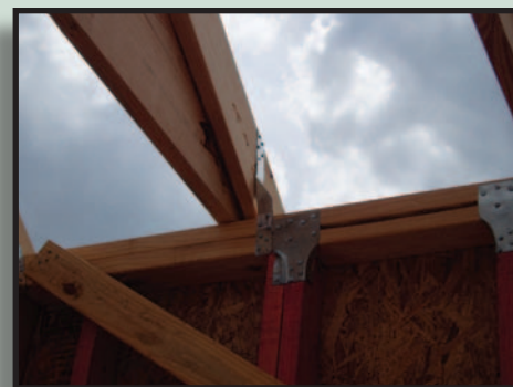
Strengthen your roof by using hurricane clips.
