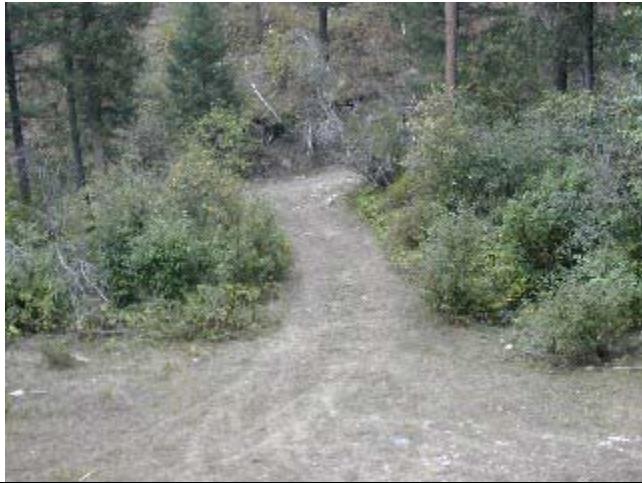
Figure 27a - Non-system road crossing of Springer Creek, before removal. August, 2006
