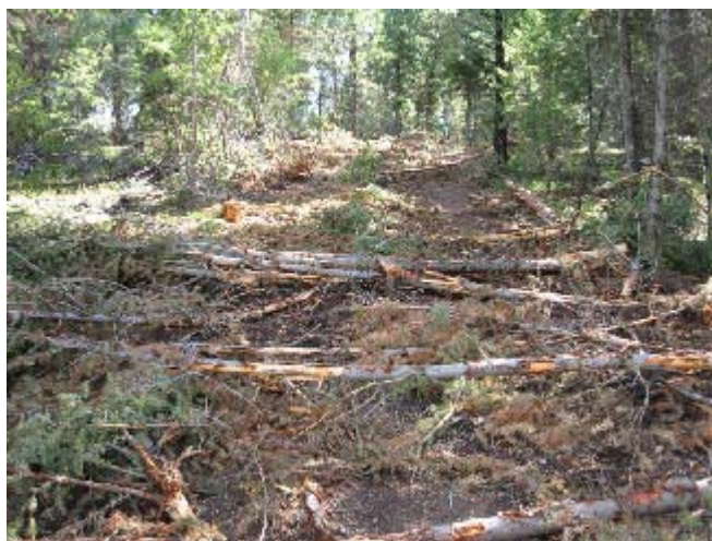
Figure 1 - Soil displacement and compaction are present where slash was not available to create a 6 to 8 inch slash mat. The slash that is present will prevent erosion. Organic and topsoil horizons are intact or slightly mixed in many locations which will maintain the native seed bank and speed natural revegetation.
