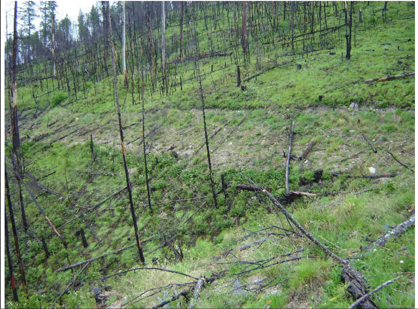
Figure 345 - Picture of obliterated Road 13326 taken in the spring of 2007. This work was completed in the Gilbert Creek Decommissioning Phase 1, 2004.
