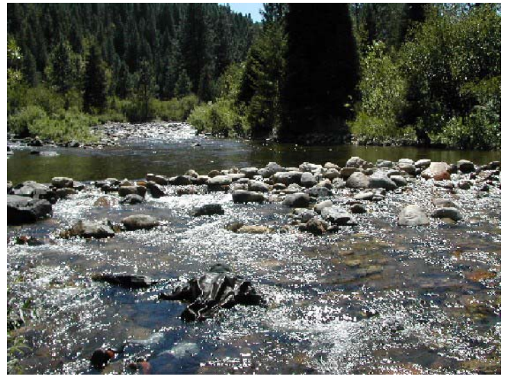
Figure 8- Rock dam in lower Running Creek. The left side of the dam was breached to allow fish passage; the right side of the photo is largely intact
