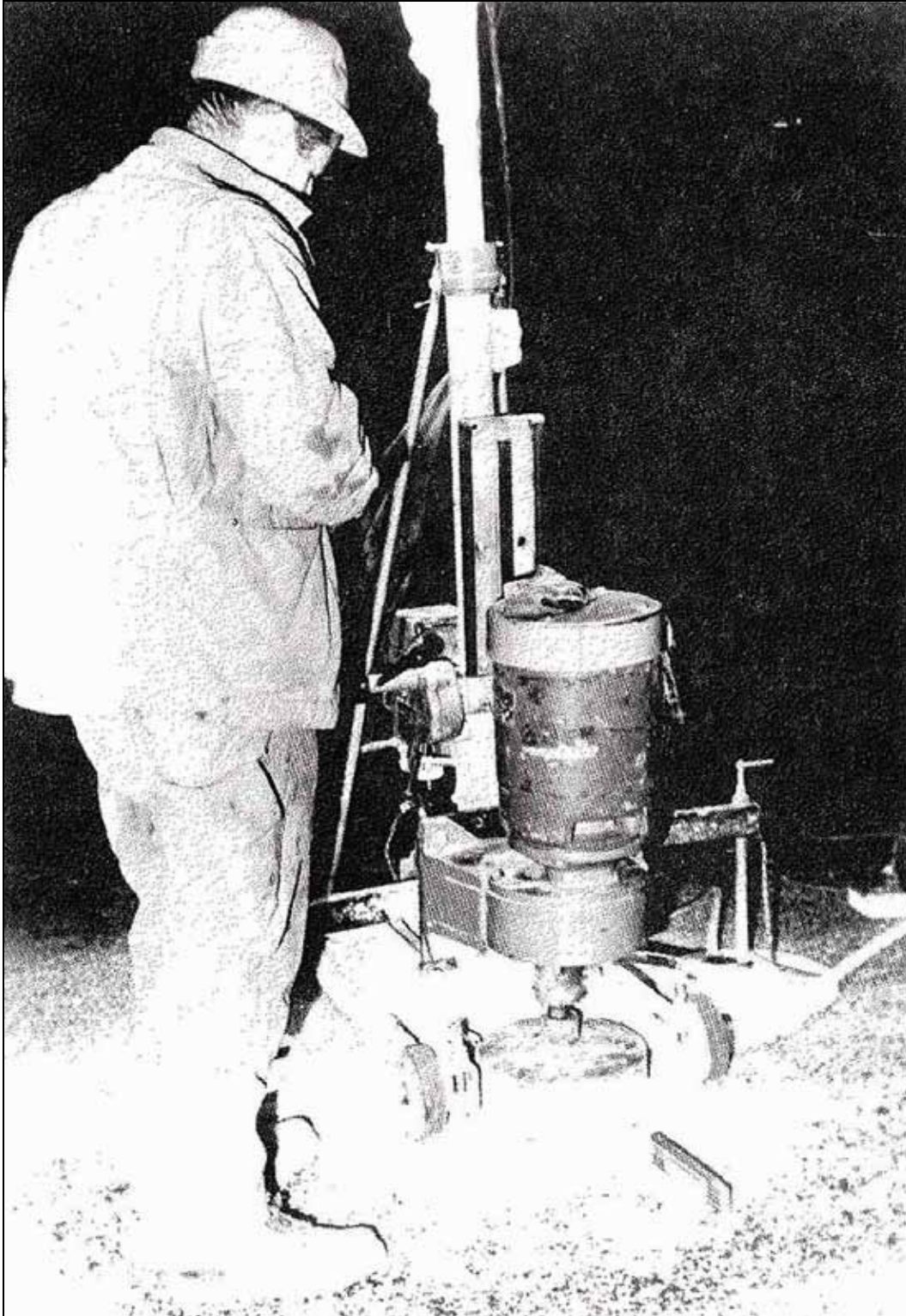
Figure 8. Core Drilling Above In-pavement Light Base (NOTE: Drilling Rig is Plumb )
