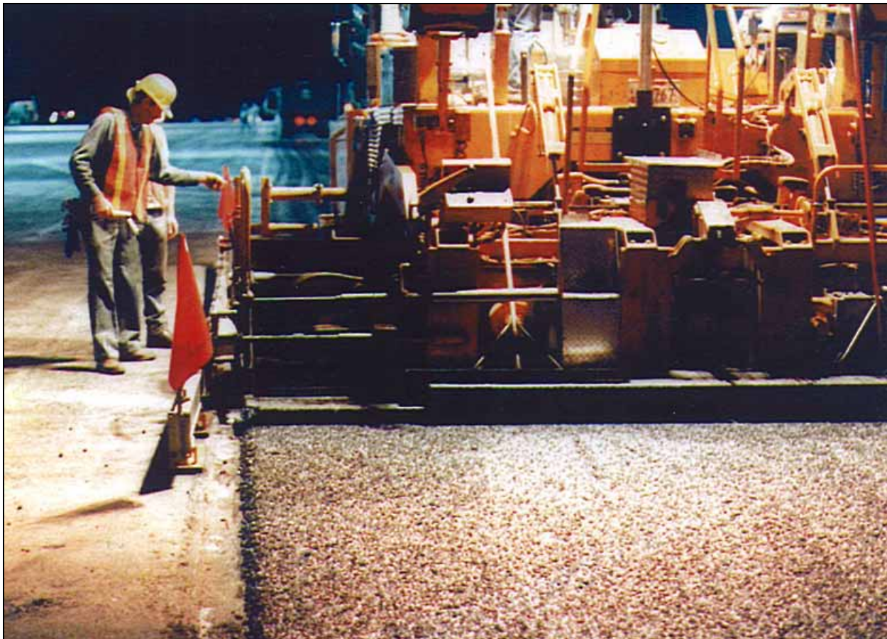
Figure 3. Pavement Spreader in Nighttime Construction
