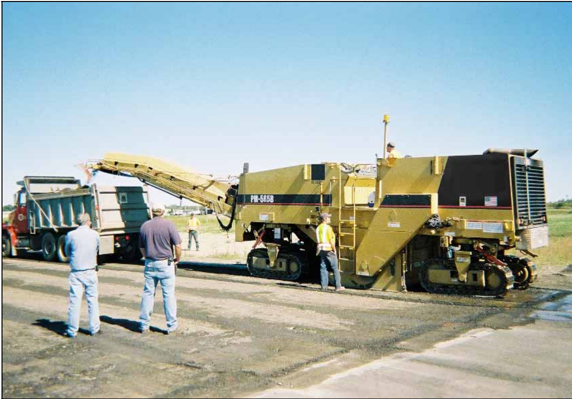
Figure 6. A Cold-Planer for Use in Removing Transition Ramp
