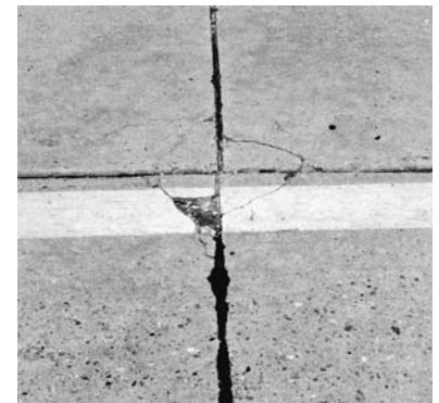
Corner cracking in all four slabs.
