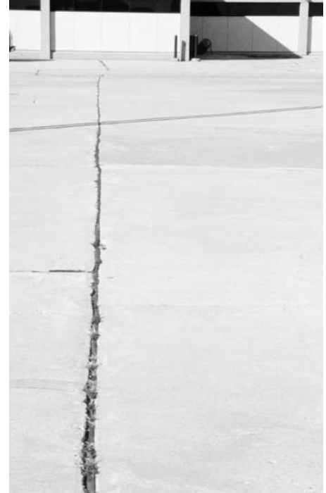
▲ Joint sealant deterioration on apron. Slab is in good condition.
