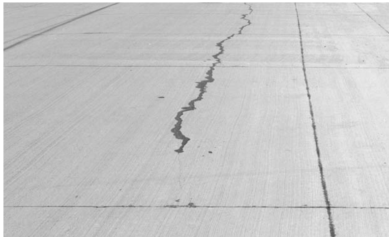
▲ Map cracking, but pavement is sound.
