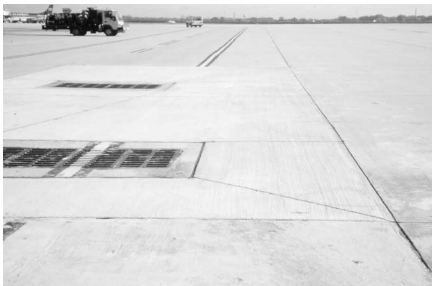
▲ Slabs replaced next to inlet. Good joint design.
