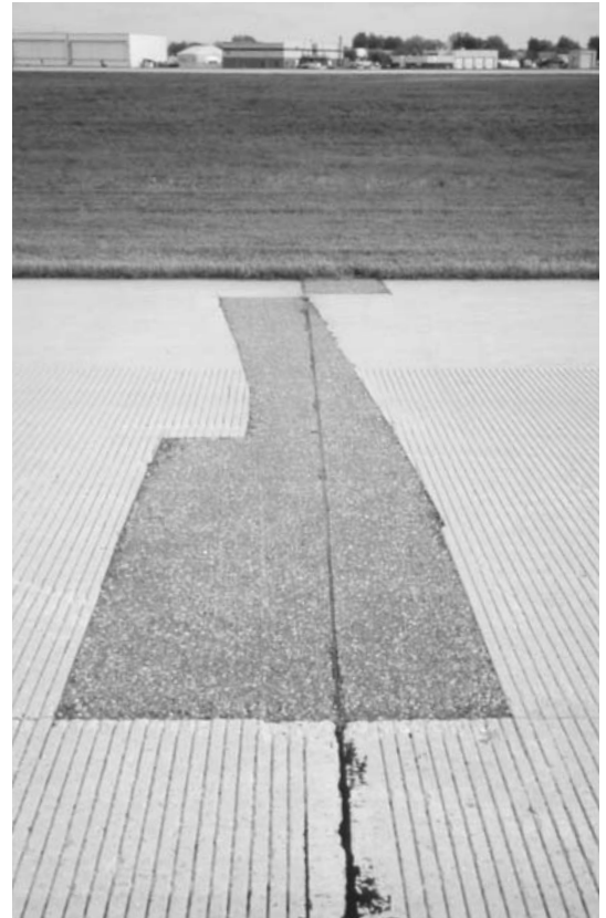
▲ Full depth joint repair. Very good condition.
