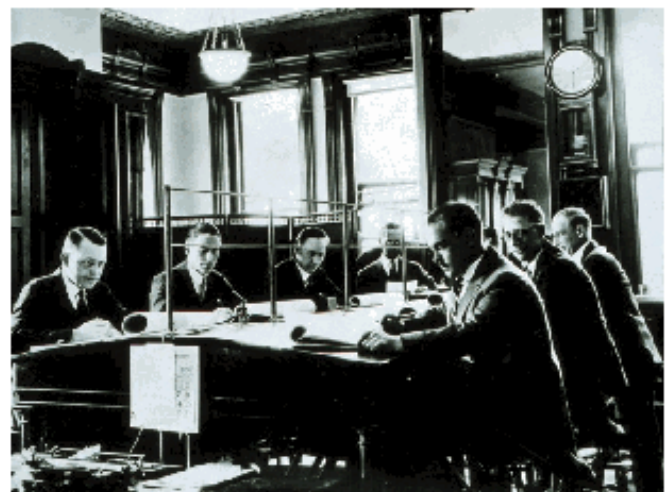
The Weather Bureau Forecast Office. Location: Washington, D.C. Photo Date: 1926
