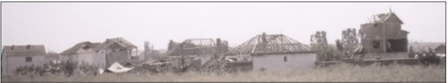
Destroyed village in southern Kosovo. This scene is typical of villages where buildings are being reconstructed this summer that were previously destroyed by Serbian forces in southern Kosovo. Photo date August 1999
