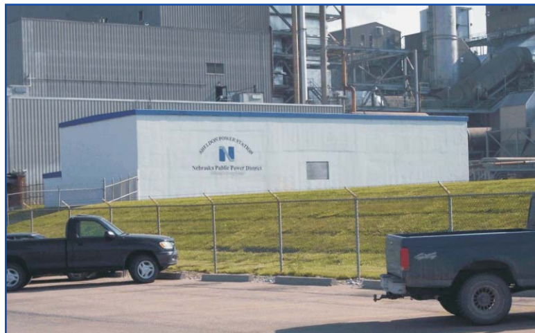
Hallam Site Intermediate Heat Exchanger Building (white building). Grassy area covers the belowground portion of the decommissioned reactor facility.
