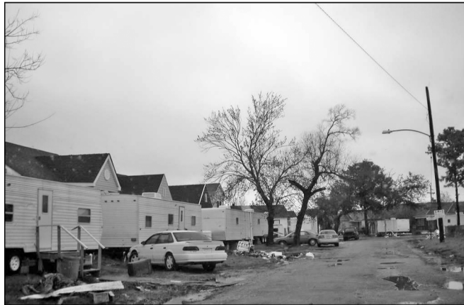
Figure 1: Trailers in Front of Damaged Housing Units in New Orleans, Louisiana
