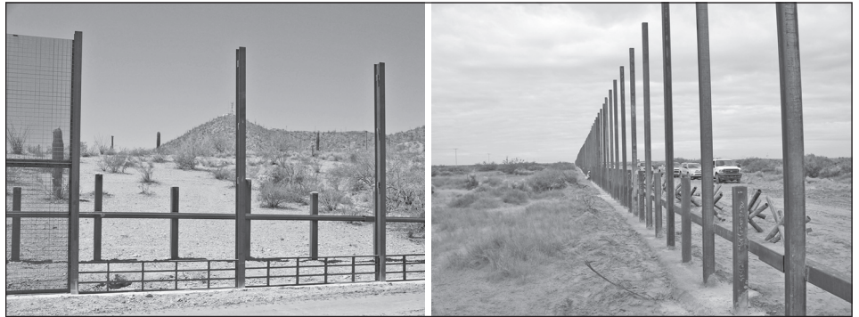
Figure 3: Examples of SBI Fence Construction
