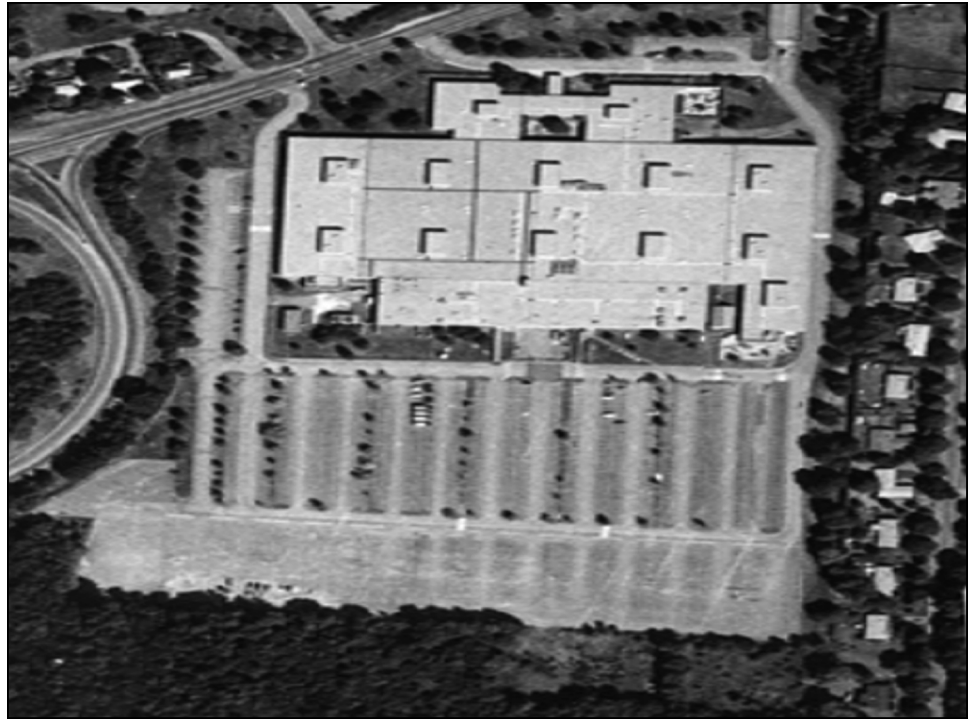
Figure 4: IRS Service Center, Andover, Massachusetts
