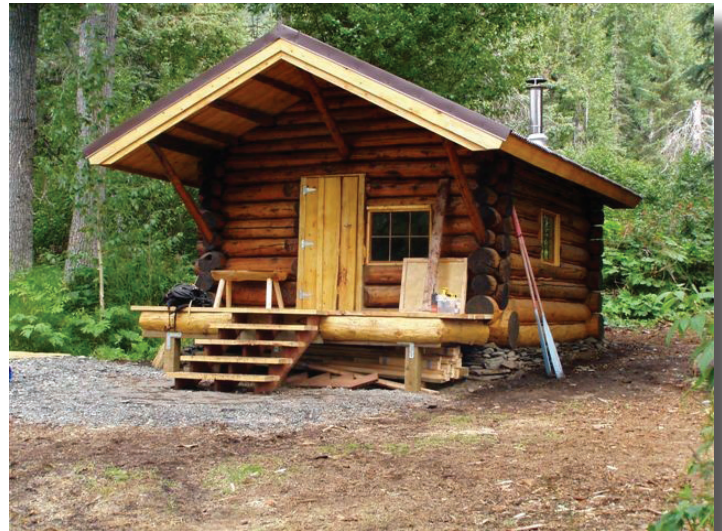
Restored historical cabin on Seward Ranger District
