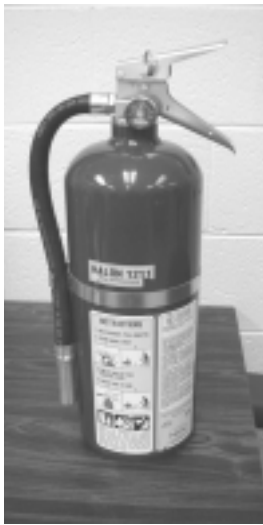
One example of halon-containing equipment. This is a hand-held Halon 1211 fire extinguisher containing a 20 lb charge. See Appendix A for a definition of halon-containing equipment. Photo courtesy of U.S. DOD/DLA ODS Reserve.
