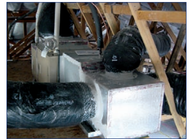
Careful sealing of air handling equipment and a sealed combustion furnace save energy and help ensure comfort and combustion safety. Placing this equipment in conditioned space improves performance.
