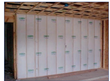
Artistic Homes uses advanced features recommended by Building America including 2-by-6-framing, allowing for R-23 blown-in insulation in the walls and R-38 in the ceiling, application of wrap and sealing to create a continuous air barrier from slab to ceiling, sealed ducts with mechanical ventilation, and transfer grilles between room for even air distribution and less drafts.
