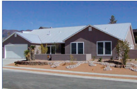
Artistic Homes of Albuquerque New Mexico built 650 homes in 2003, all of them using Building America principles.
