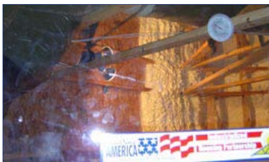
Shoppers love to peer into the attic through this viewing window in a Building America model house by Cambridge Homes. Shoppers can see the special insulation, and the thermometer tells them how cool the attic stays.
