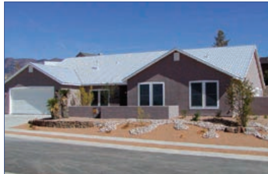
Artistic Homes of Albuquerque New Mexico built 650 homes in 2003, all of them using Building America principles.
