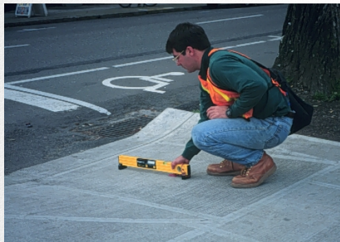
Figure 11-17. The curb ramp slope is being measured for positive slope with a digital inclinometer.
