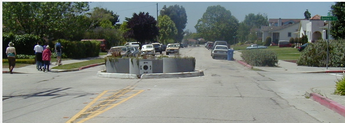
Figure 9-17. Neighborhood traffic circles are a common horizontal measure for controlling the speed of motorists at a low volume intersection.
