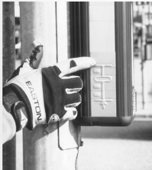
Figure 6-14. GOOD DESIGN: In addition to providing audible and vibrotactile information, Swedish pedestrian signals include a simple tactile map of the pedestrian crossing. This intersection has a median and three lanes of traffic.
