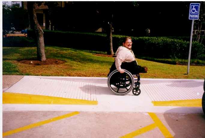
Figure 7-37. Parallel curb ramps work well on narrow sidewalks but require users continuing on the pathway to negotiate two ramp grades.
