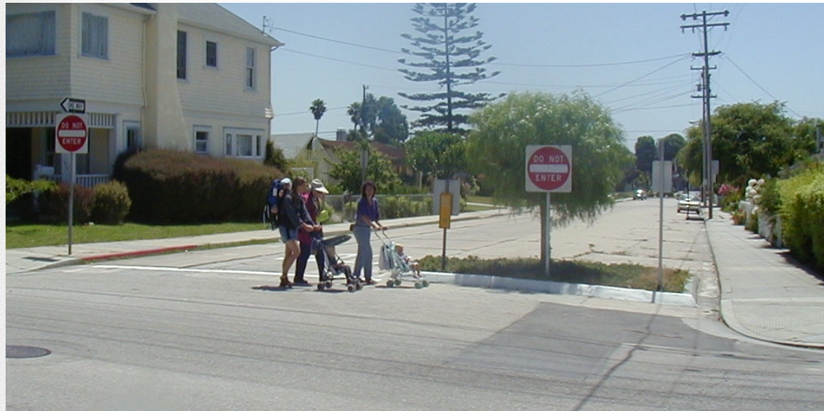
Figure 9-1. Half closures placed at intersections are a traffic calming technique intended to divert motorists off of residential streets by closing one-half the roadway and allowing one-way traffic. Half closures reduce crossing distances for pedestrians.
