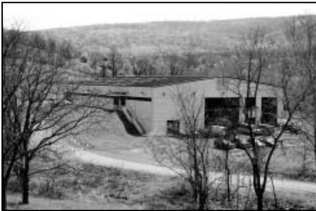
Canine Training Facility in Front Royal, VA.
