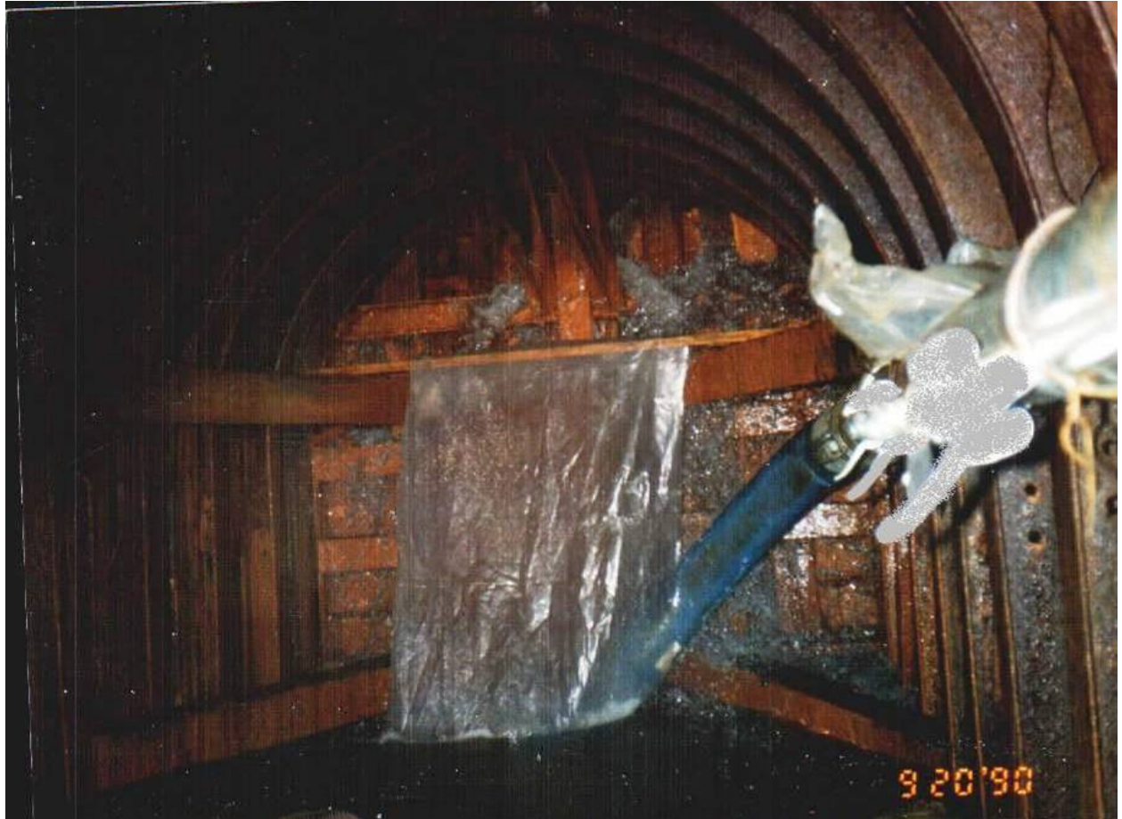
Figure 6. Bulkhead at Station 4+66 (date noted on photo)
