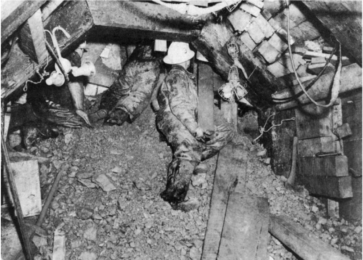
Figure 5. Running Ground in the Parting quartzite (approximate date August/September 1951)
