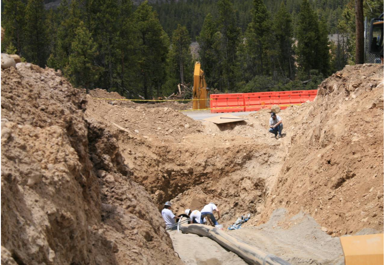
Figure 8. Excavation into the Glacial Moraine at Leadville for installation of a pipeline under Highway 91 along the alignment of the LMDT (late spring 2008)
