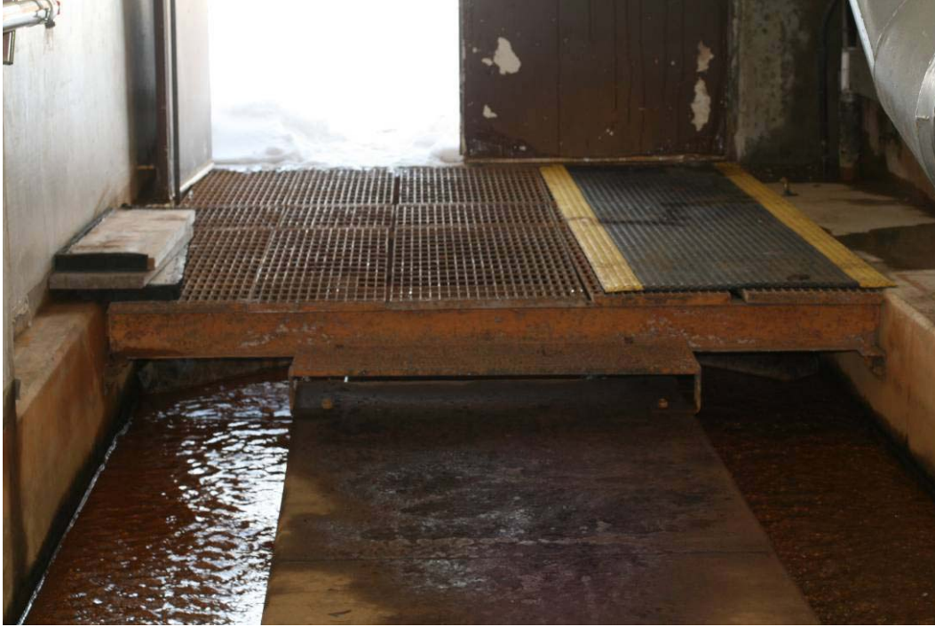
Figure 18. Photograph taken on March 25, 2008 looking at the downstream end of the LMDT showing the concrete center walkway with drainage ditches on either side and steel floor grating.
