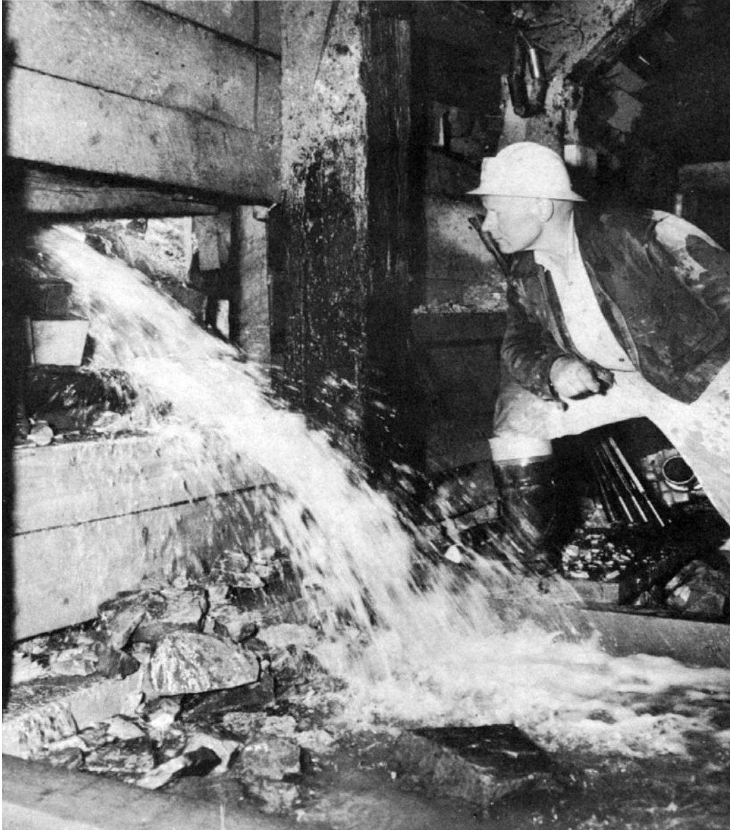
Figure 12. Photograph showing the inflow to the LMDT through a drillhole connected to the Robert Emmet shaft, taken from (Salsbury, 1956). This is prior to driving the Robert Emmet lateral.
