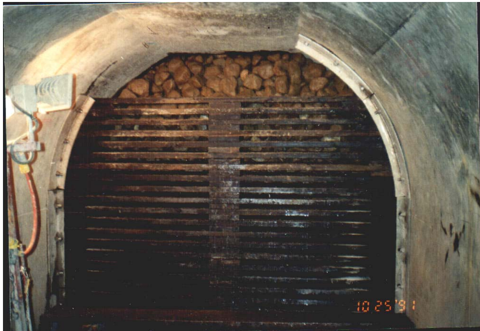
Figure 26. Construction photograph showing the cobbles behind the timber-lattice bulkhead at Station 4+60 of the LMDT.
