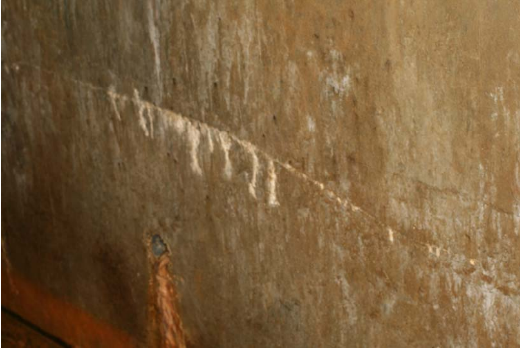
Figure 21. This crack located about 3 feet above the LMDT floor is the only one that showed offsetting of the concrete. The offset is about 1/8 inch.
