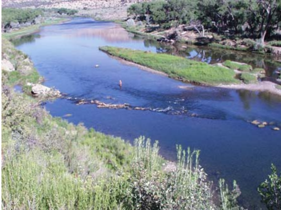
Cottonwood Diversion and Intake Gallery.
