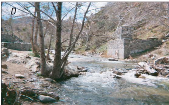
Big Rock Creek gaging station, San Gabriel Mountains near Valyermo (10263500; March 2004). Channel is bedrock; width about 3 m. High flow is from snowmelt.
