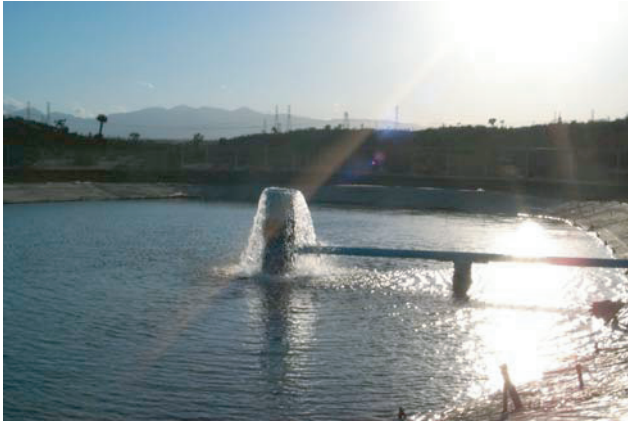
Figure 17. Photograph of artificial recharge pond along Oro Grande Wash, western Mojave Desert, southern California. Flow from standpipe is about 50 liters per second.
