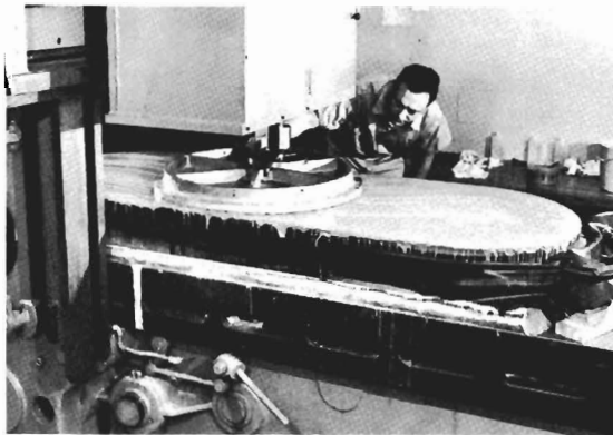
Grinding and polishing of glass.
