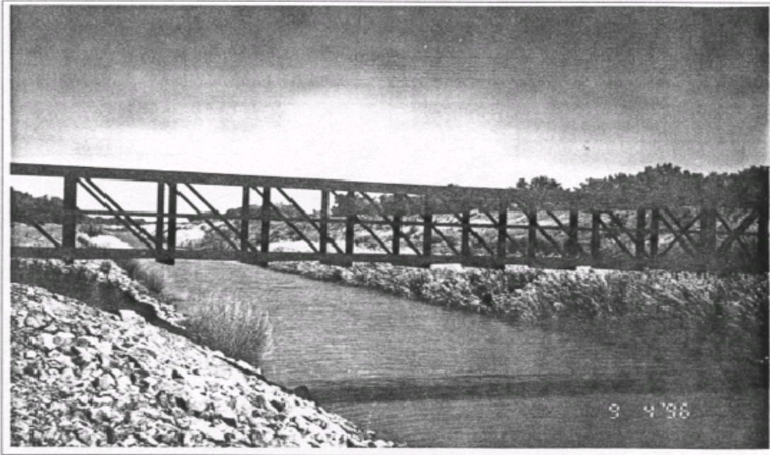
BRIDGE ABOVE SEDIMENT SAMPLING STATION
