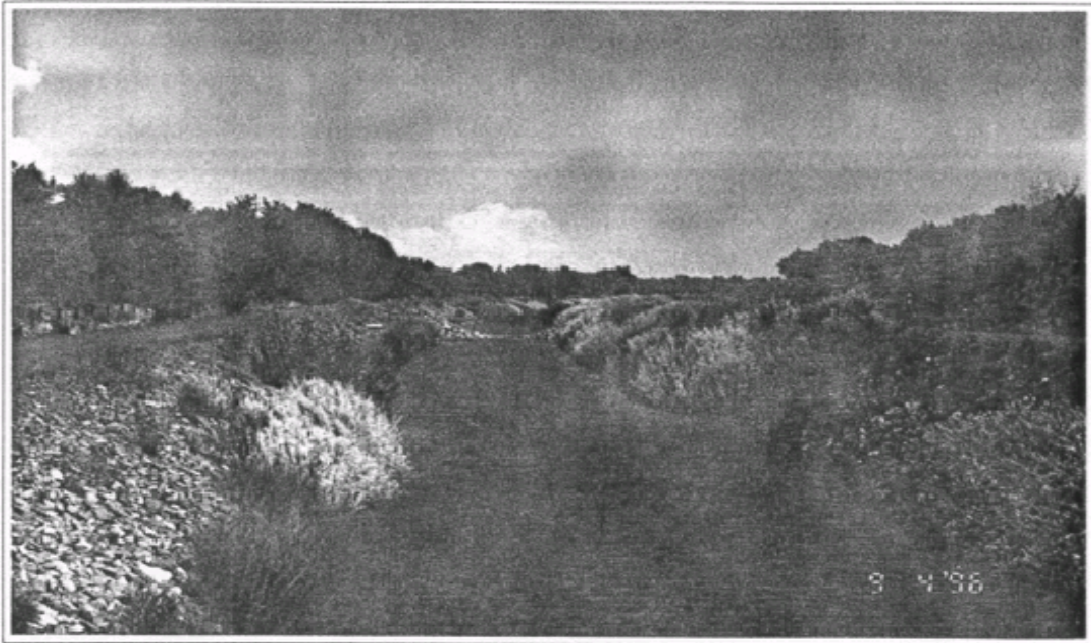
GRADE CONTROL STRUCTURE
