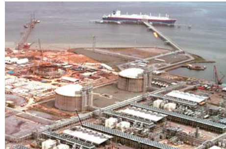
After liquefaction, the LNG is stored in insulated tanks until it can be loaded onto carrier ships. This photo shows such tanks in Trinidad and Tobago.
