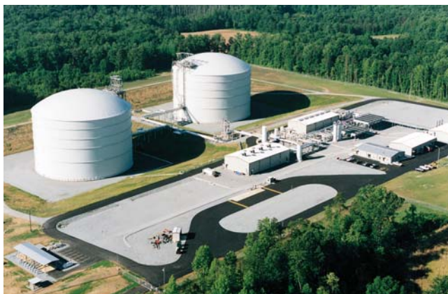
The Pine Needle, North Carolina peak-shaving facility, one of the largest in the nation, has a storage capacity of 4 Bcf. A sendout capacity of .4 Bcfd empties the tanks in 10 days of peak usage.
