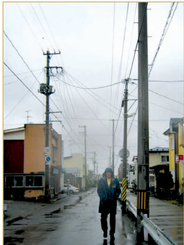
figure 8. Hachinohe street showing parallel public and private distribution feeders.
