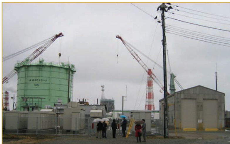
figure 10. Central generation facility at the Hachinohe water treatment plant.
