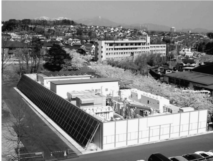
Figure 6: Sendai microgrid installation. (source: NTT Facilities)
