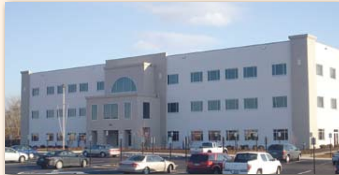
Newly constructed leased facility for the U.S. Coast Guard National Maritime Center in Martinsburg, West Virginia
