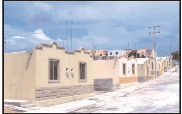
Prefabricados y Modular de Monterrey (PyMM) will use a $10 million OPIC loan to help Mexico meet a growing demand for low-income housing.
