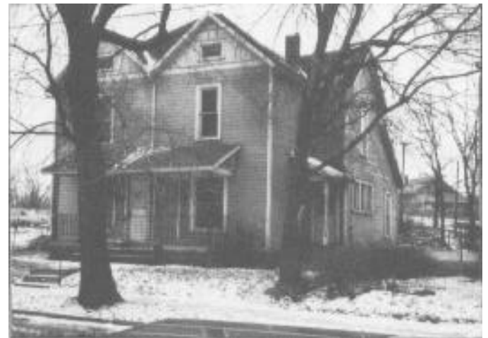
158 Eureka Street--slated for rehabilitation and candidate for fire sprinkler project.
