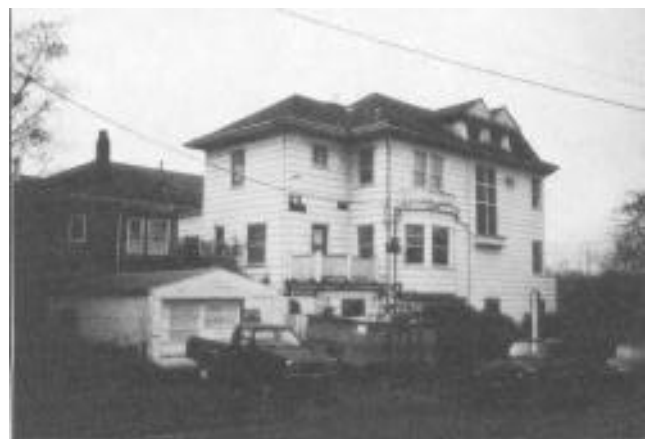
Victoria Apartments, Seattle, WA, Rear View
