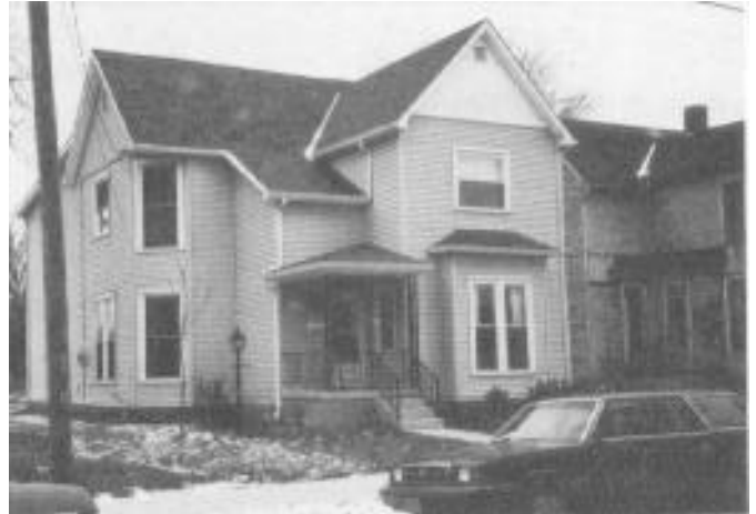
157 Eureka Street--After Rehabilitation.
