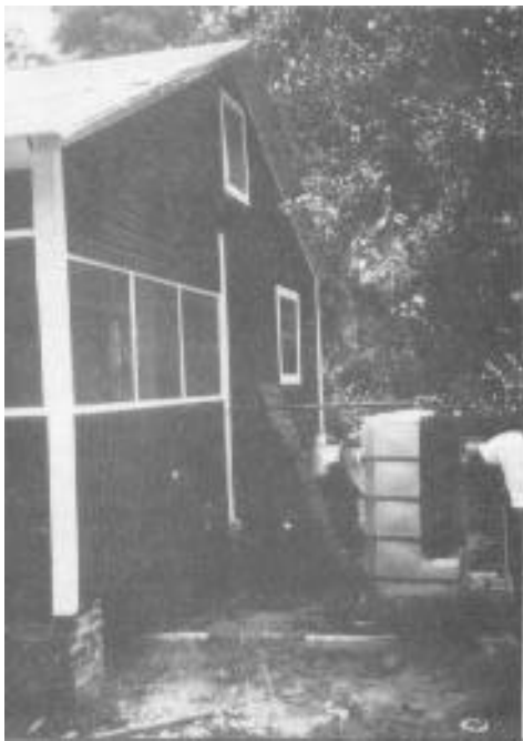
Pump and reservoir system, located behind house.
