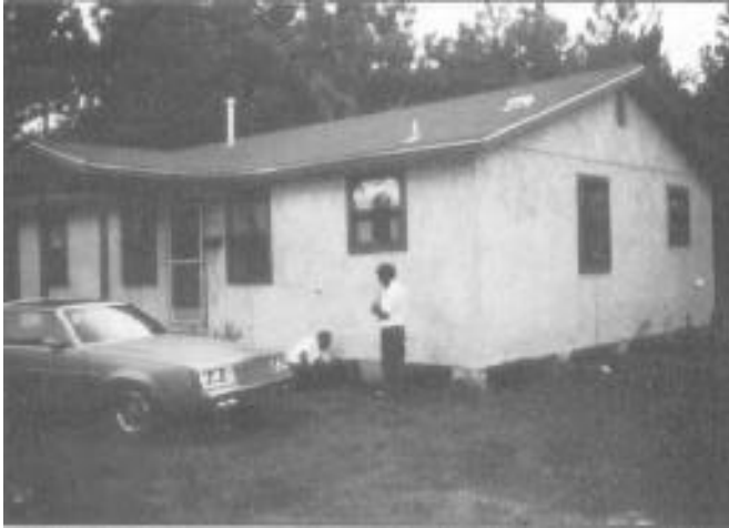
Sprinklered House at 1448 Miller St., Orange Park, FL.
