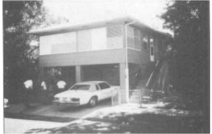
Sprinklered House at 1040 11th Street South
