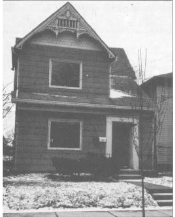
120 Eureka Street--slated for rehabilitation and candidate for fire sprinkler project.
