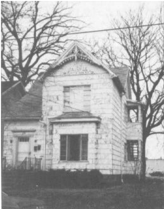
119 Eureka Street--slated for rehabilitation and candidate for fire sprinkler project.
