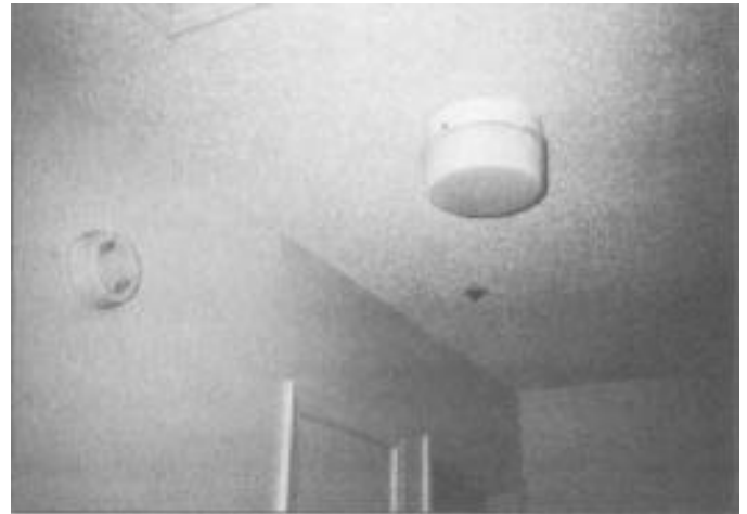
819 Seventh Avenue, Quincy, Interior View
