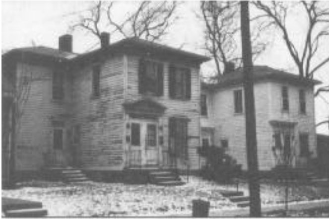
114 Eureka Street--slated for rehabilitation and city of Lima's "parade of Homes," a public relations campaign focused on rehabilitated homes.
