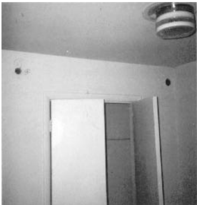
Holes for sprinkler piping through finished walls.
