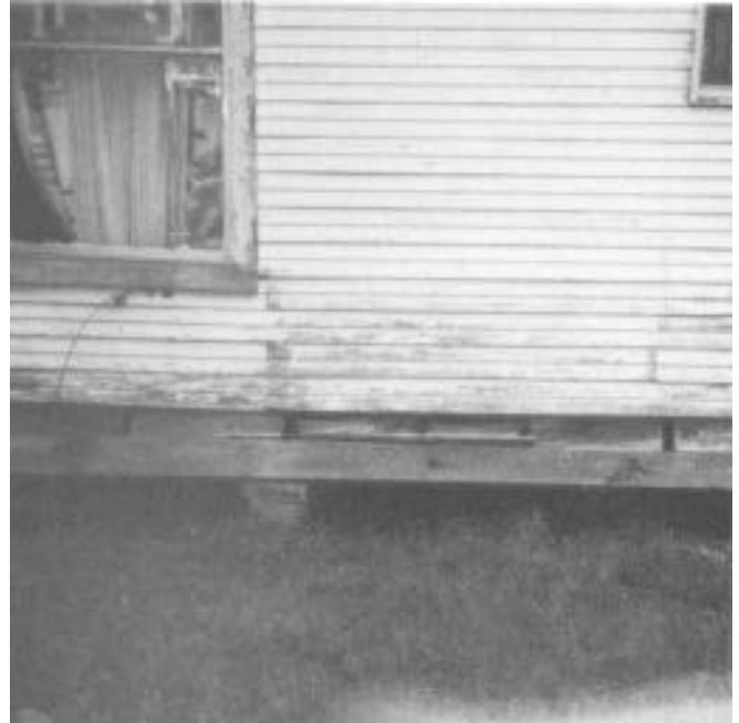
Foundation of 3501 Pennsylvania Avenue.
