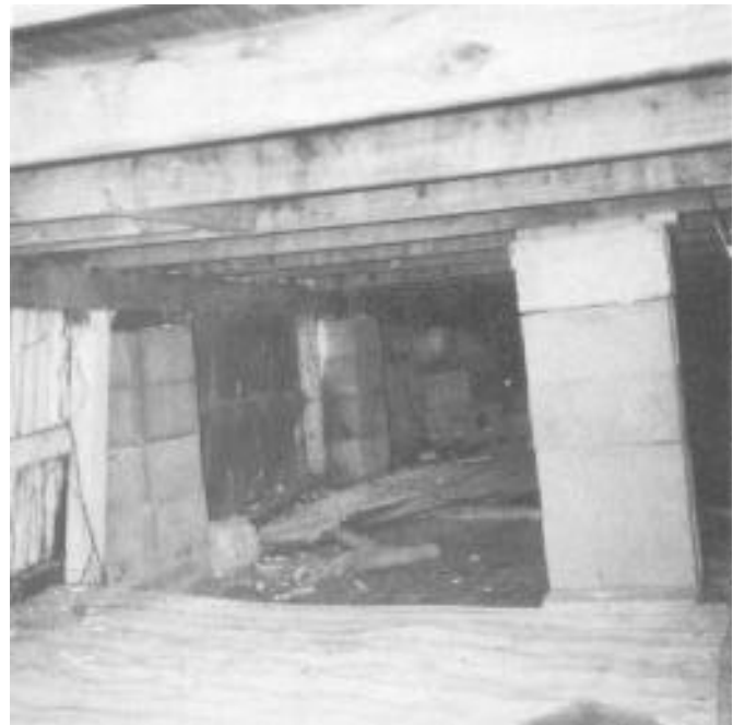
Underside of 3501 Pennsylvania Avenue Prior to Skirting.
