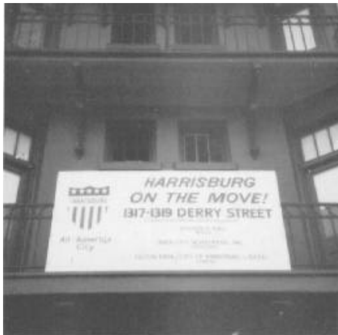
Exterior view of 1317/19 Derry Street.
