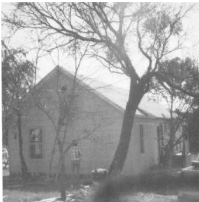
Contractors working on exterior of 3501 Pennsylvania Avenue.
