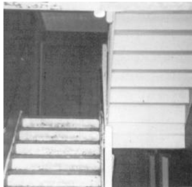
Common interior stairway at 5353 Sheriff Road.
