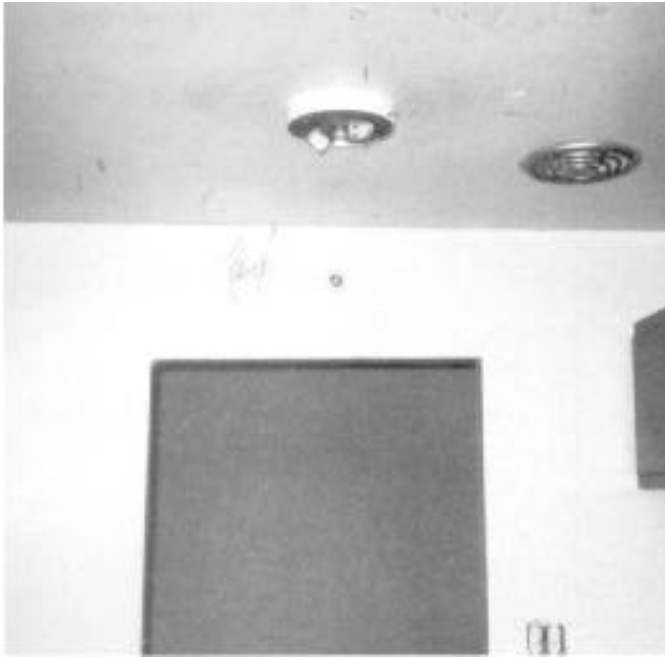
Sidewall head in finished rehabilitated kitchen.
