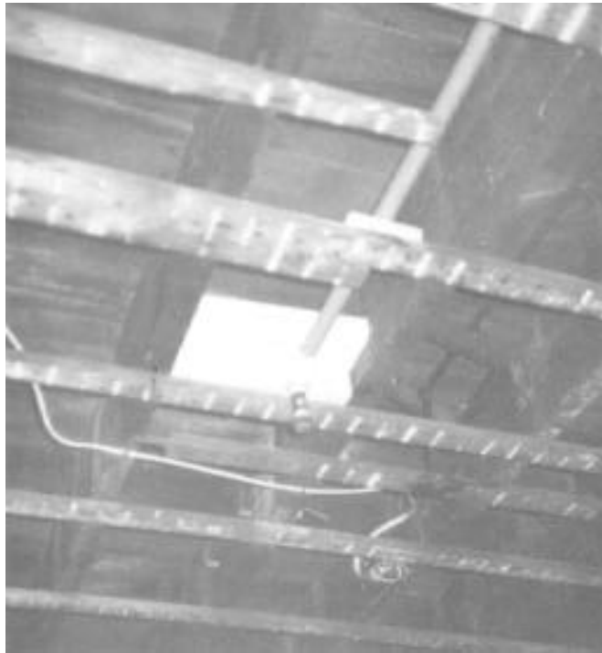
Blocking in joists for sprinkler head connection.
