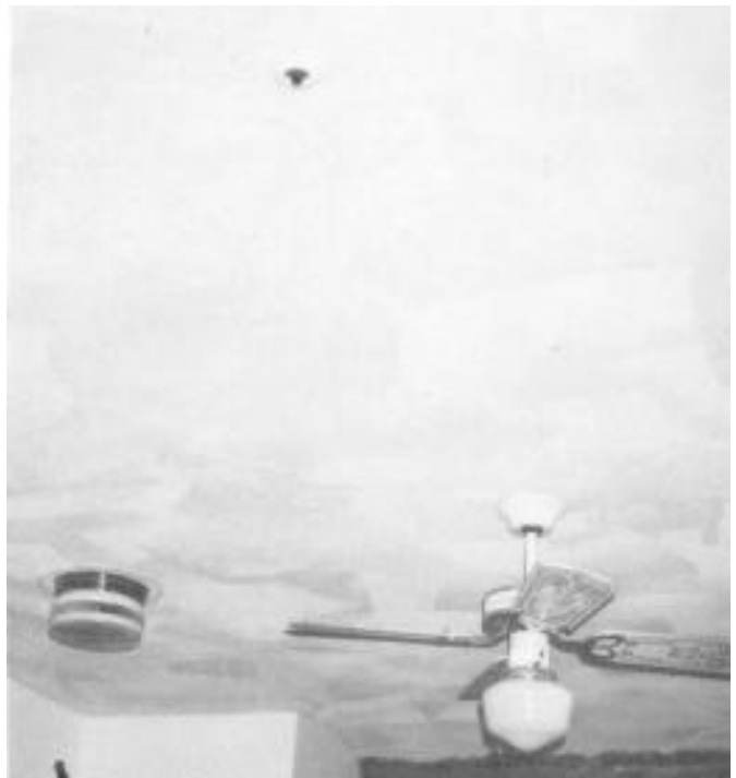
View of finished units.
