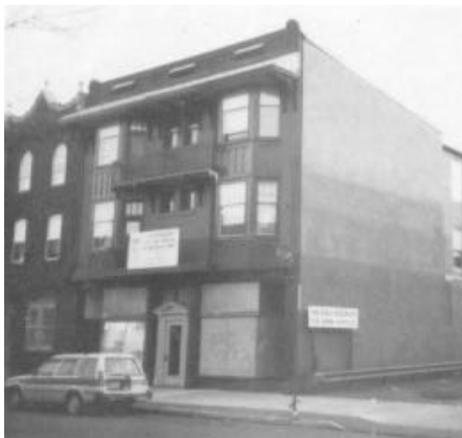
Exterior view of 1317/19 Derry Street.
