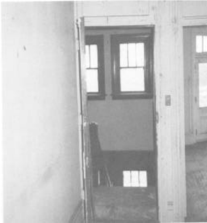
View of interior prior to rehabilitation.
