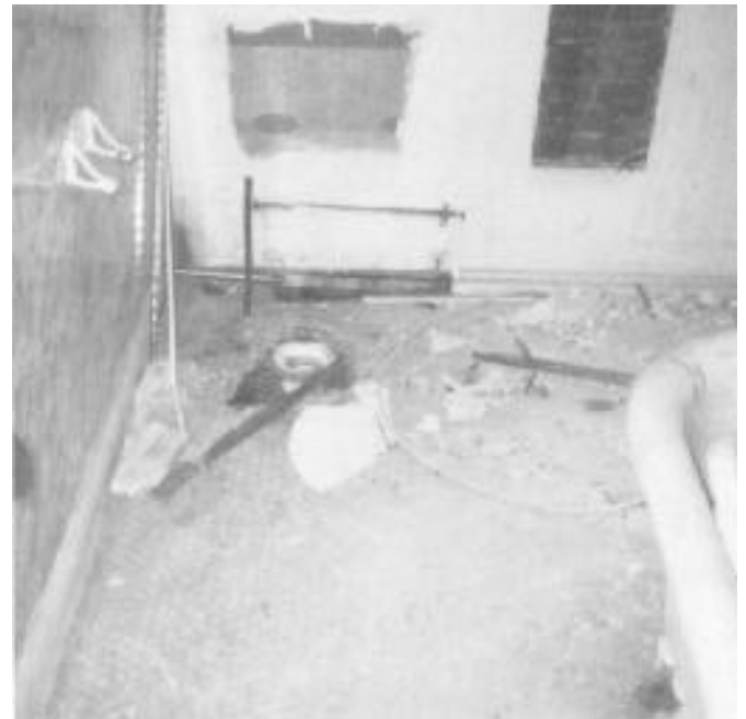
View of Interior prior to rehabilitation.
