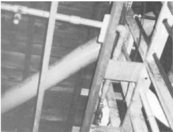
Adjacent water systems--domestic and sprinkler during rehabilitation.
