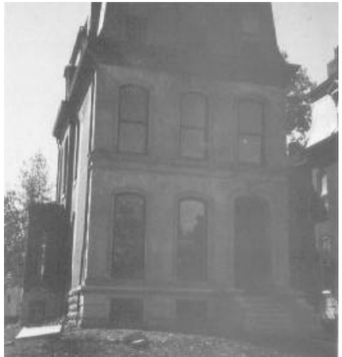
Frontal view of 2102 Lafayette Avenue prior to rehabilitation.
