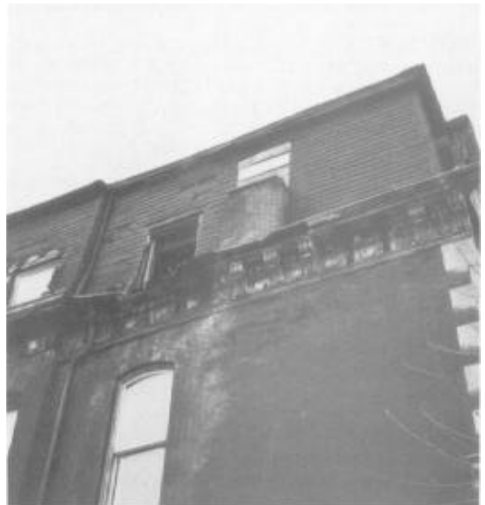
Side view prior to rehabilitation.
