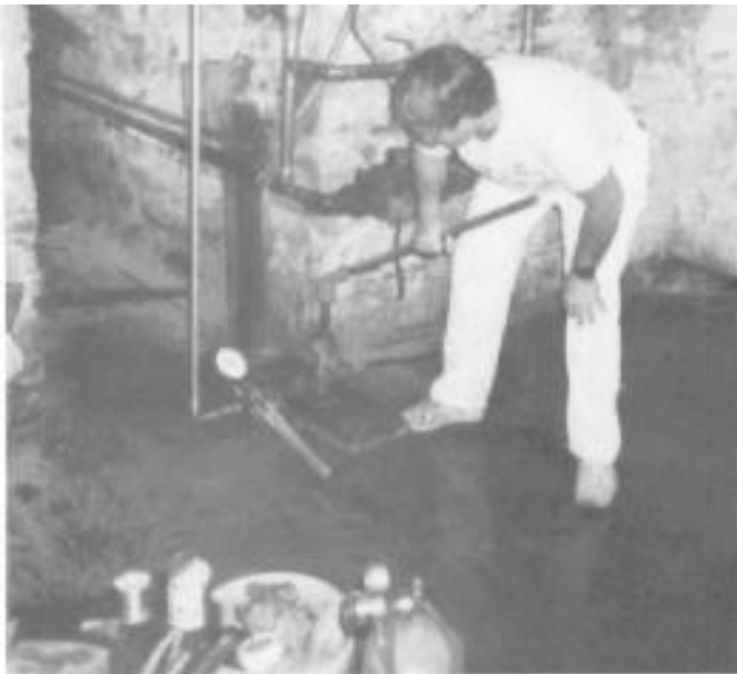
Mr. Hal Lanshe pumping system to 203 PSI by hand.
