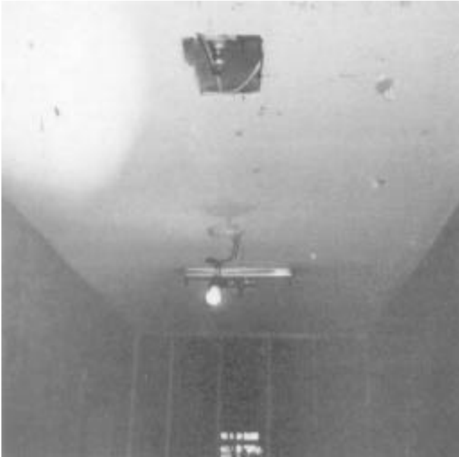
Sprinkler head connection through nearly complete ceiling.
