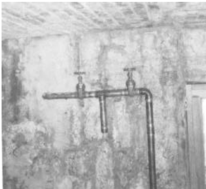
Old water system prior to rehabilitation.
