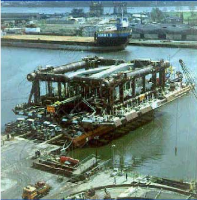
Load-out in Rotterdam
