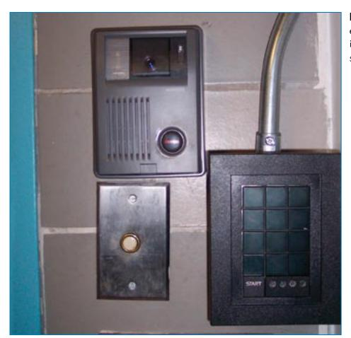
Figure 5-7: Electronic entry control device into restricted area.
