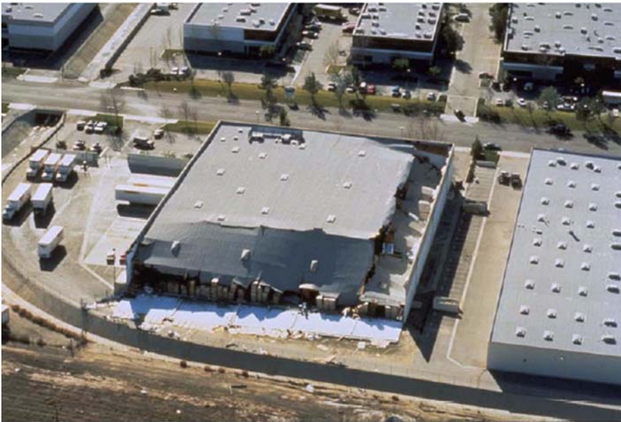
Figure 8-1 Roof and wall collapse of tilt-up building during the 1994 Northridge earthquake. (Photo courtesy of the Earthquake Engineering Research Institute)
