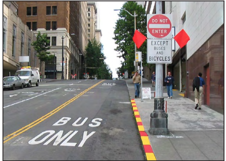
Speed and Reliability developed a contra-flow lane on Seneca Street between Second and Third avenues to provide faster, more reliable access to Third Avenue for buses coming off the Alaskan Way Viaduct.
