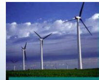
NSP 107 MW Lake Benton, MN wind farm
