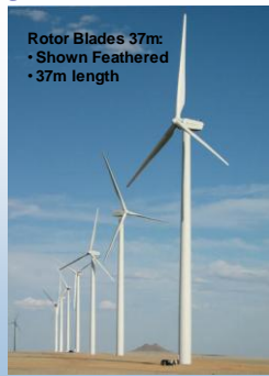
A Utility Scale 1.5 MW Wind Turbine
