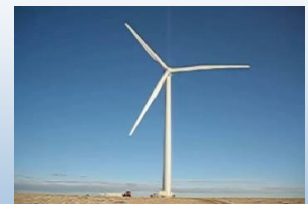
93 Meter Diameter and 2.5MW
