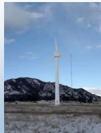
15 Meter Diameter and 100 kW
