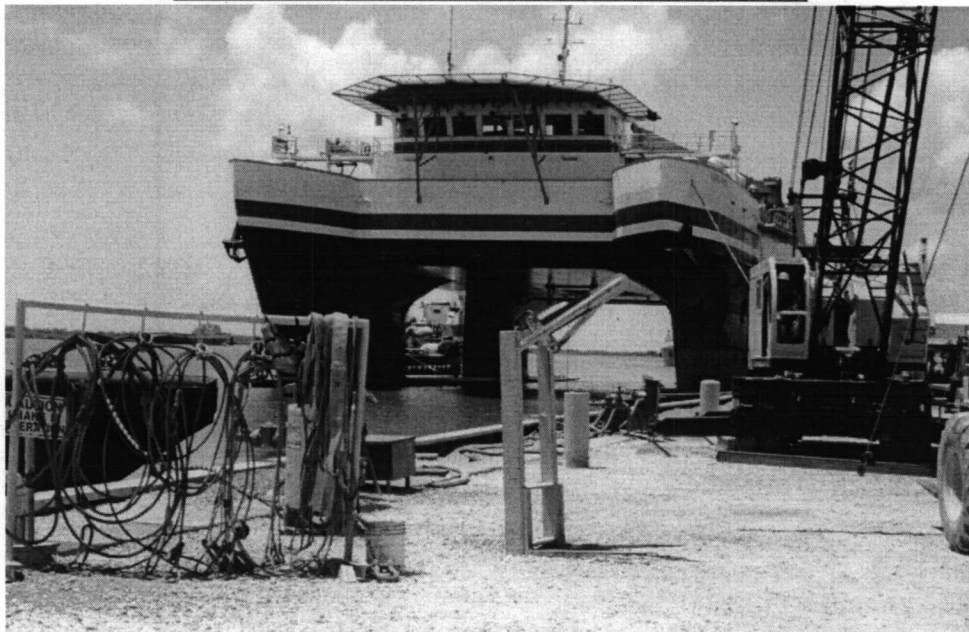
Figure 4. Large vessels requiring a deeper draft can be accommodated at Port Fourchon. The increased activity in deepwater oil and gas activities has made the port vitally important to industry.
