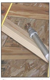
This sprinkler should be located at least 10.5 inches (270 mm) from the truss web.
