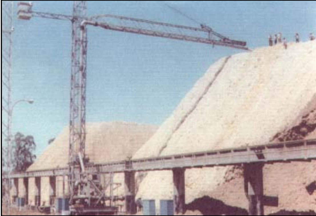
Figure 3.1 Wet Storage Pile Construction
