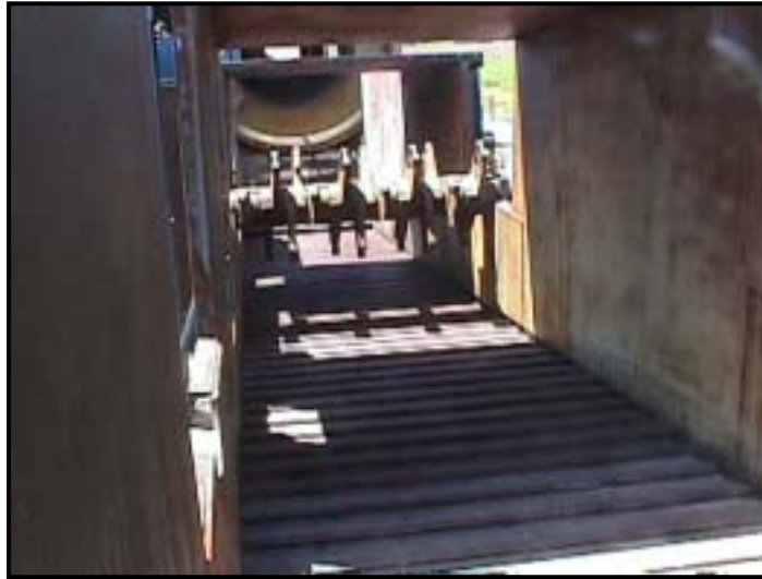
Figure 12 7'x7' Interior of Washer
