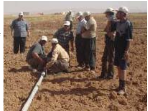
Staff from the Ministry of Agriculture lay lateral pipes during the practical training portion of the course.
