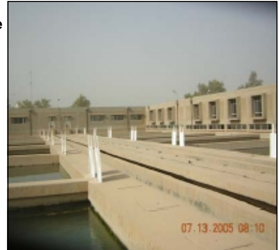
USAID's refurbished water treatment plants will treat approximately 90 million gallons of water per day.
