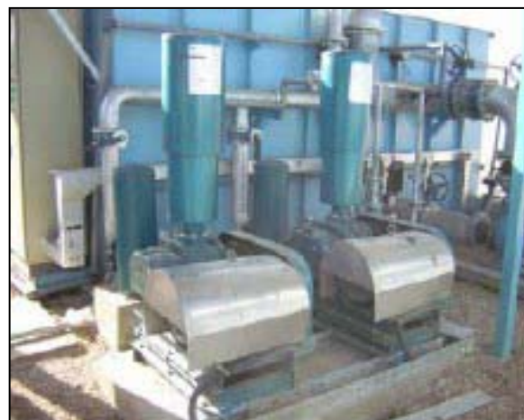
Restored Basrah water treatment facilities.
