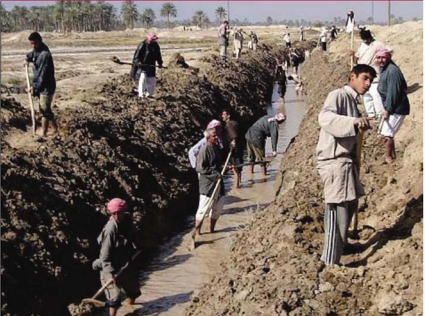
Cleaning the canals of weeds and silt will improve the flow of water and drainage to reduce salinity in agricultural areas. USAID has recently completed a grant to clean canals in the Muthanna Governorate, restoring much of the local irrigation infrastructure.
