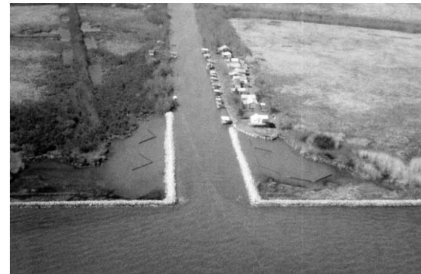
In addition to high-altitude aerial photography, DNR also obtains low-altitude images. This shot shows the Boston Canal-Vermilion Bay Shoreline Stabilization Project after the installation of rock breakwaters along Boston Canal. (DNR photo)
