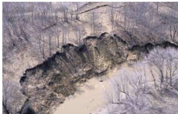
Example of streambank erosion in Missouri. (Photo courtesy of USDA NRCS)
