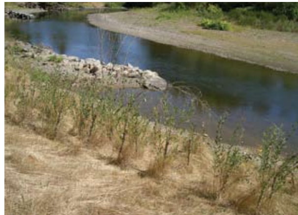
Streambank stabilization with stream barbs and riparian re-vegetation in Oregon. (Photo by K. Boyer, USDA NRCS)
