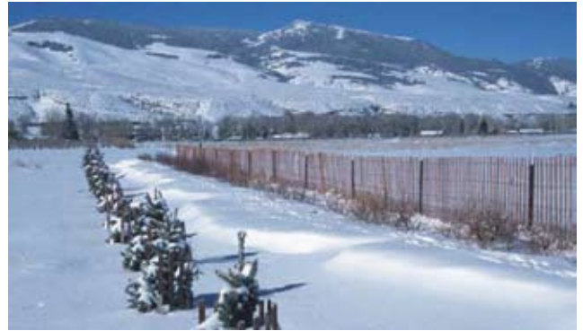
Living snow fence designed to control snow deposition. (Photo courtesy of USDA NRCS)
