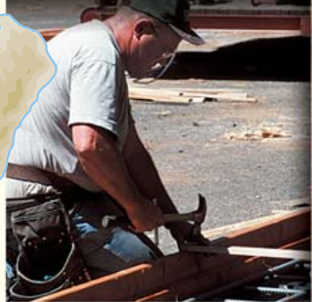
Shore Acres State Park entrance rebuilt
