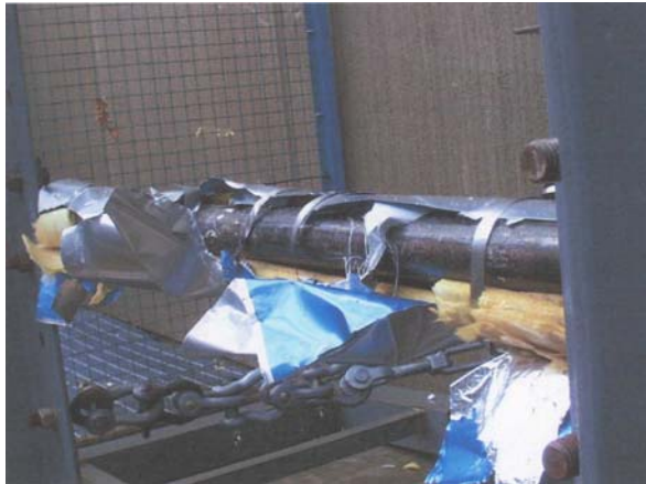
Back side of target pipe
