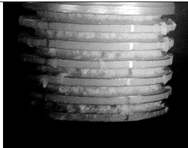
Accumulation of a small amount of fiber between fins of a stacked-disk strainer
