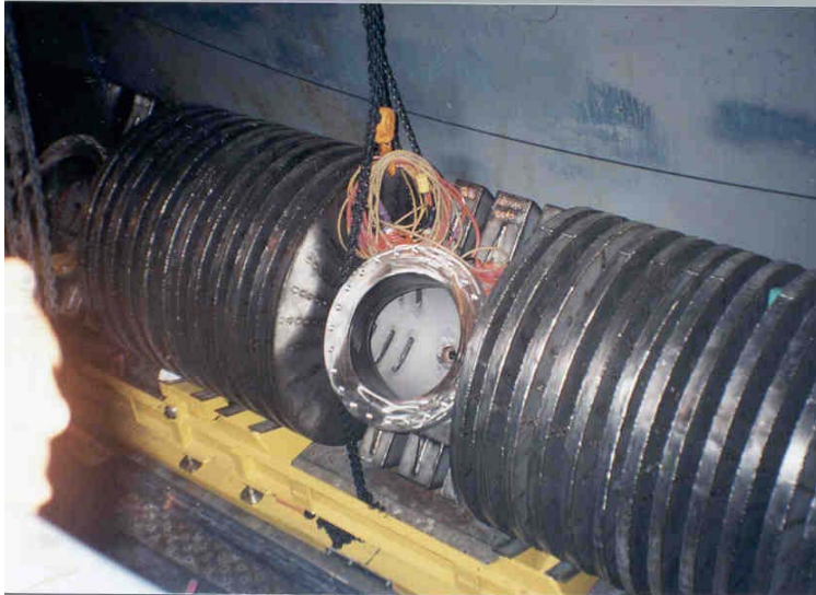
Figure 8-3 PCI Stacked-Disk Strainer Being Installed at Pilgrim Nuclear Power Plant
