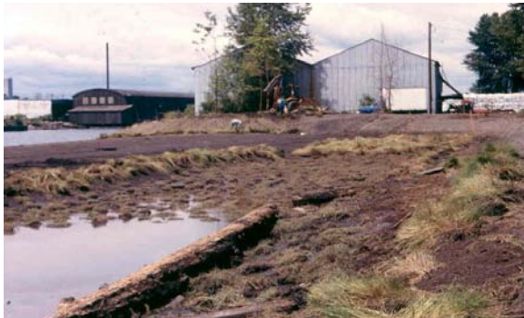
Photo 24 June 1995 Salvage in progress
