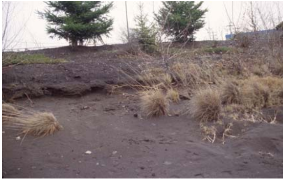
Photo 20 January 2003 Erosion @ base of berm
