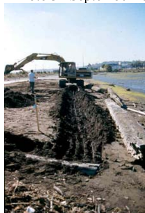
Photo 33 September 1999 Log placement
