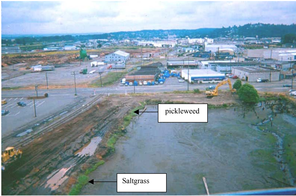
Photo 11 Construction June 1995 (photo courtesy Simpson)
