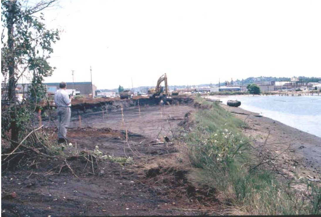
Photo 7 Construction of North Peninsula 1995
