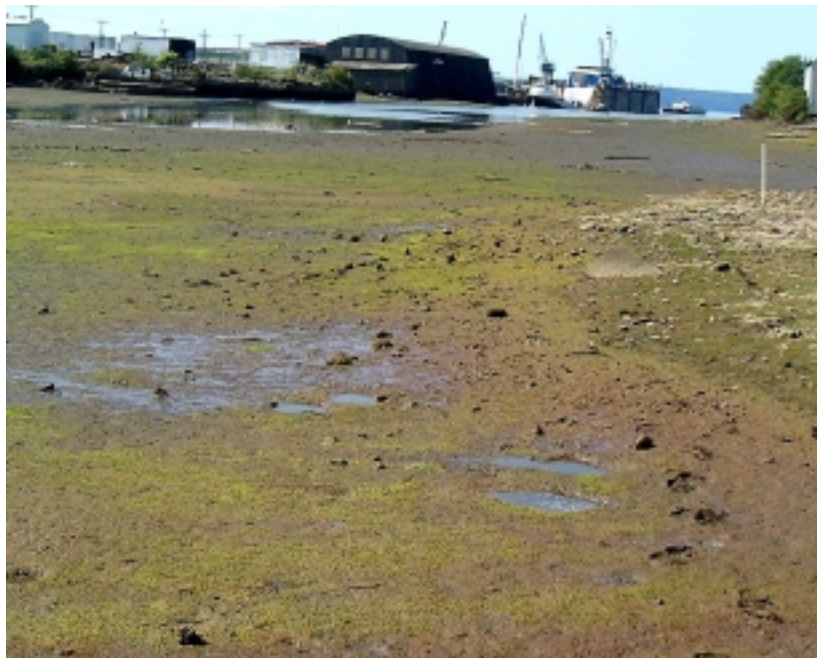
Figure D-14. View North towards Waterway Inlet (8/1/00)
