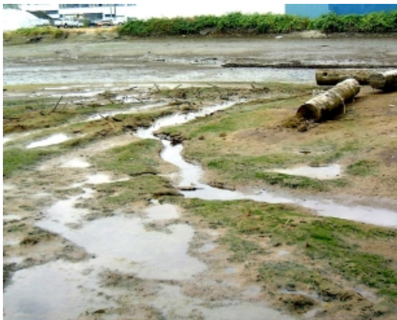
Figure D-10. Channel Forming South of Berm (Looking southwest, 8/1/00)
