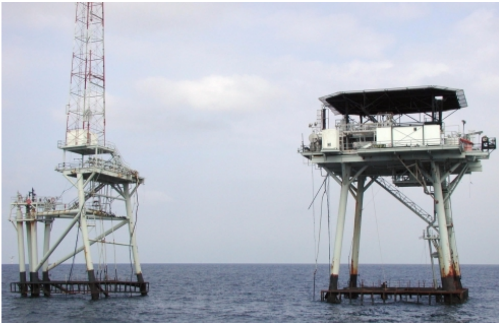
EI-231-CA is on the left. This is a post-storm photo and the bridge that used to connect the two facilities was destroyed in the storm.
