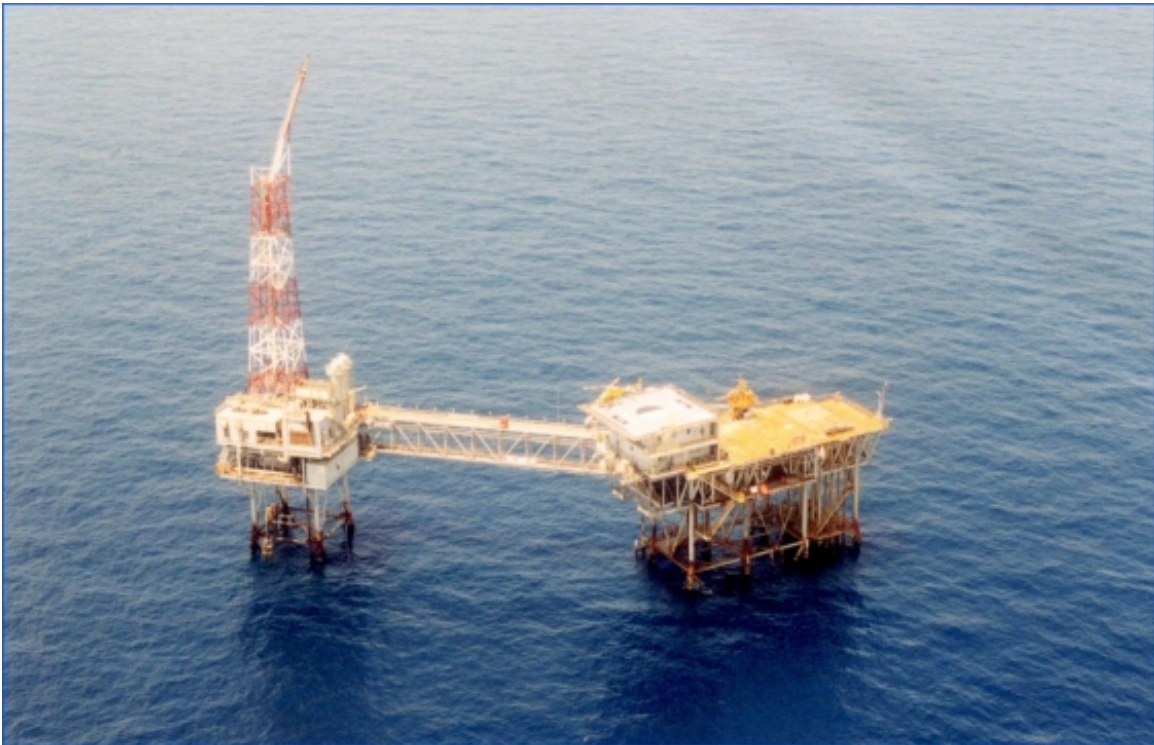
EI-295-A-PRD is shown in a pre-storm photo on the left. The drilling platform is on the right.
