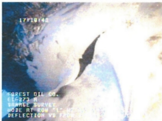
NODE AT ROW 1, HZ A1B1 AT -130', DEFLECTION AND TEAR IN VD FROM B1 @ -75'
