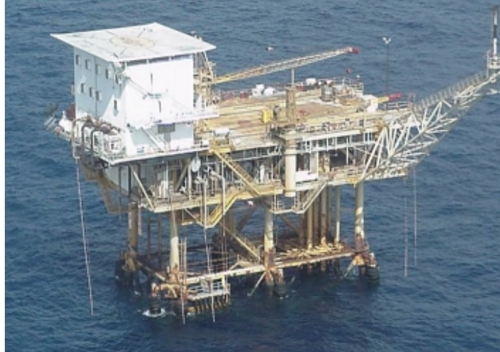
EI-337-A shown in a pre-storm photograph.
