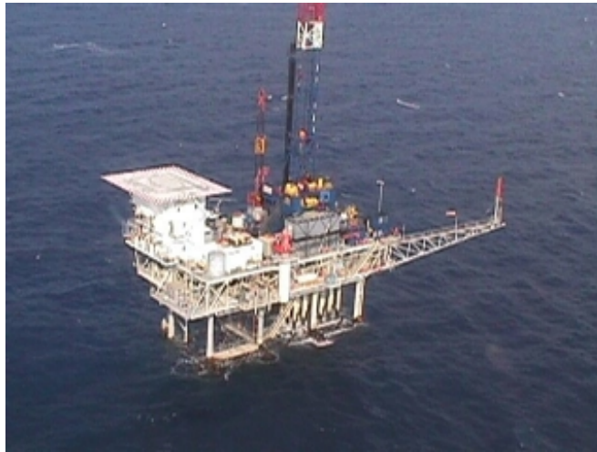
EI-330-B shown in a pre-storm photograph.
