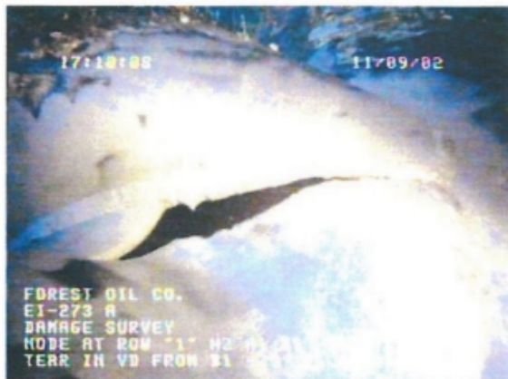
NODE AT ROW 1, HZ A1B1 AT -130', DEFLECTION AND TEAR IN VD FROM B1 @ -75'
