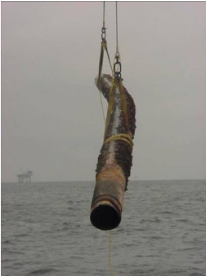
Figure 6– Global Buckle of Brace. Picture taken during removal.
