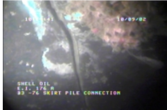
Damage to EI-276-A-VALVE identified during subsea inspections at connections between the skirt piles and the main jacket
