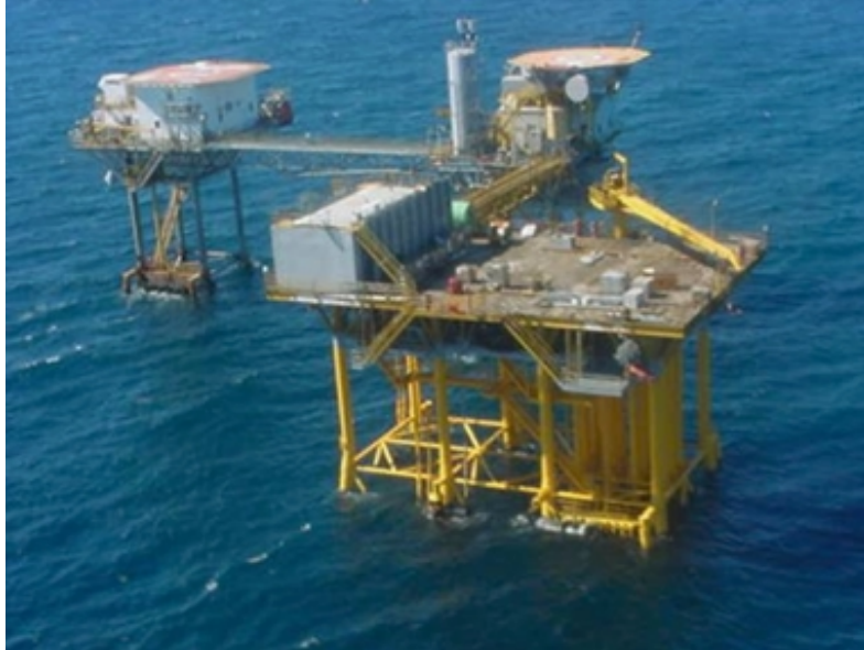
EI-276-B-Aux shown in the rear left of this photo before Hurricane Lili
